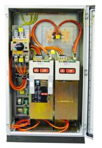
Complete engineered welding control in self contained easy to install cabinet, safety screens, circuit breaker with door interlocking, optional isolation contactor, power supplies and earth leakage protection.
