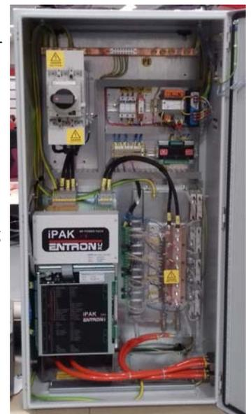
Example: Complete iPAK 600A system with 4 transformer outputs.
