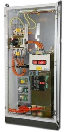
Control fitted into a sheet steel enclosure with circuit breaker, 24 VDC air valve power supply, appropriate line fusing, safety covers, and water-cooled MFDC Inverter Module. Optional hand-held pendant.
